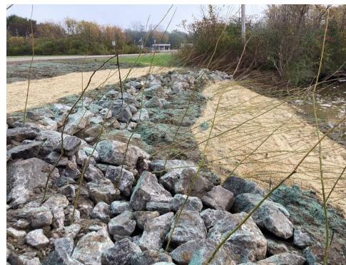
In 2021, CWC assisted the Town of North Harmony in writing a successful grant application to fund work to stabilize a creek bend threatening Stow Road and to create a larger functioning flood plain to store stormwater and dissipate stream energy to reduce stream bank erosion downstream. CWC also assisted with native plant selections for the project. This was one of several erosion control and restoration projects completed on Ball Creek with assistance and guidance from CWC.
